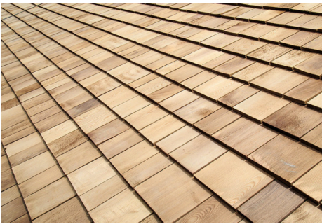
CEDAR SHINGLE ROOF
